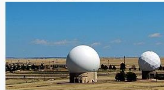
Radome installations at Schriever
